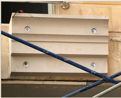
Cornice detail — installed roofline component
