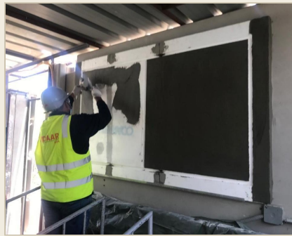
On-site application — same-material finishing
